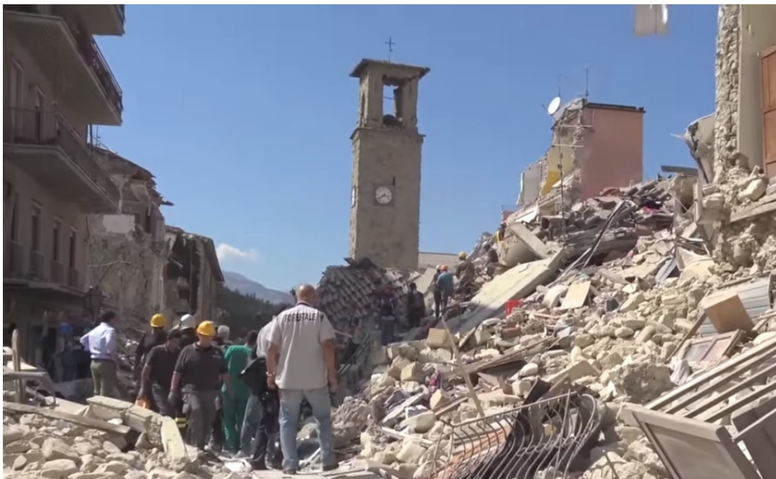
Figure 3.21: The town center of Amatrice Italy after the August 24 th 2016 earthquake that measured 6.2 on the moment magnitude scale; note that the bell tower (lower natural frequency) is still standing while shorter stiffer structures (higher natural frequency) have suffered extensive damage. a
