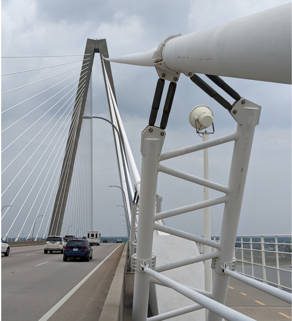
The Arthur Ravenel Jr. Bridge spans the Cooper River outside of Charleston South Carolina (USA) with a main span of 471 m (1,546 feet) and uses dampers on the center cables to mitigate wind and traffic-induced vibrations in the structure. It is the third longest among cable-stayed bridges in the Western Hemisphere (2023).
